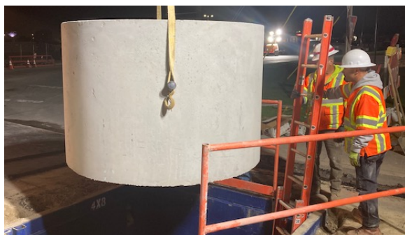
Crews lowering a concrete cylinder to reinforce the manhole shaft.
