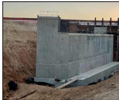
Crews constructing the bridge support system, called abutments, for the new Van Buren Boulevard bridge.
