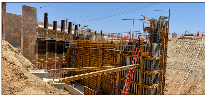
Crews constructing the bridge support system, called abutments, for the new Van Buren Boulevard bridge.
