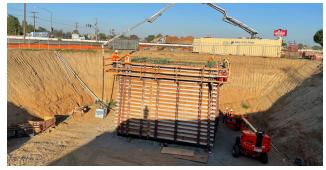
Nearly 276-cubic yards of concrete were placed for the storm water pump station wet well walls. When complete, these concrete walls extend 40 feet below finish grade.
