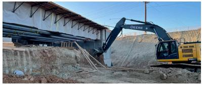
Crews are excavating dirt near the Van Buren Boulevard bridge support system to lower Jurupa Road 26 feet. Jurupa Road will ultimately go under the new Van Buren and UPRR bridges.
