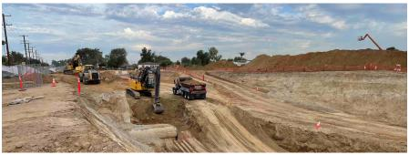
Crews excavating dirt to lower Jurupa Road west of the Van Buren Boulevard bridge. This dirt will be transported to backfill the Storm Water Pump Station wet well area east of Van Buren Boulevard at Felspar Street.
