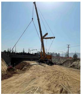
Looking east on Jurupa Road to the very beginning stages of the new Van Buren Boulevard bridge where this crane placed six of the 12 large, 17,000 pound concrete girders for the bridge support system.
