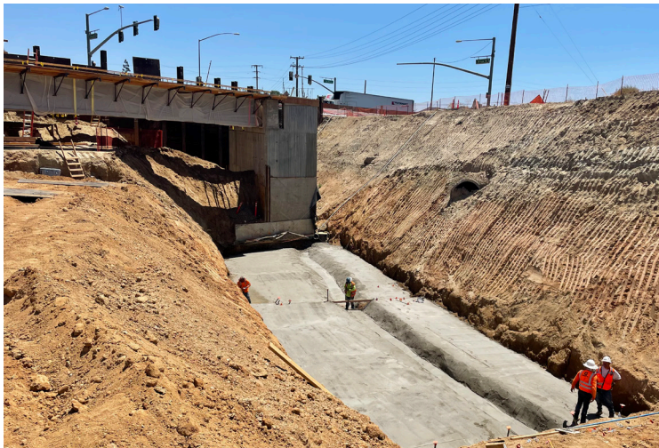
Crews working on the future retaining wall system where the lowered Jurupa Rd. will be constructed.
