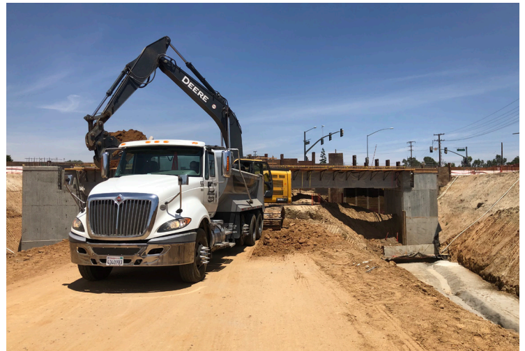
Crews working on the future retaining wall system where the lowered Jurupa Rd. will be constructed.
