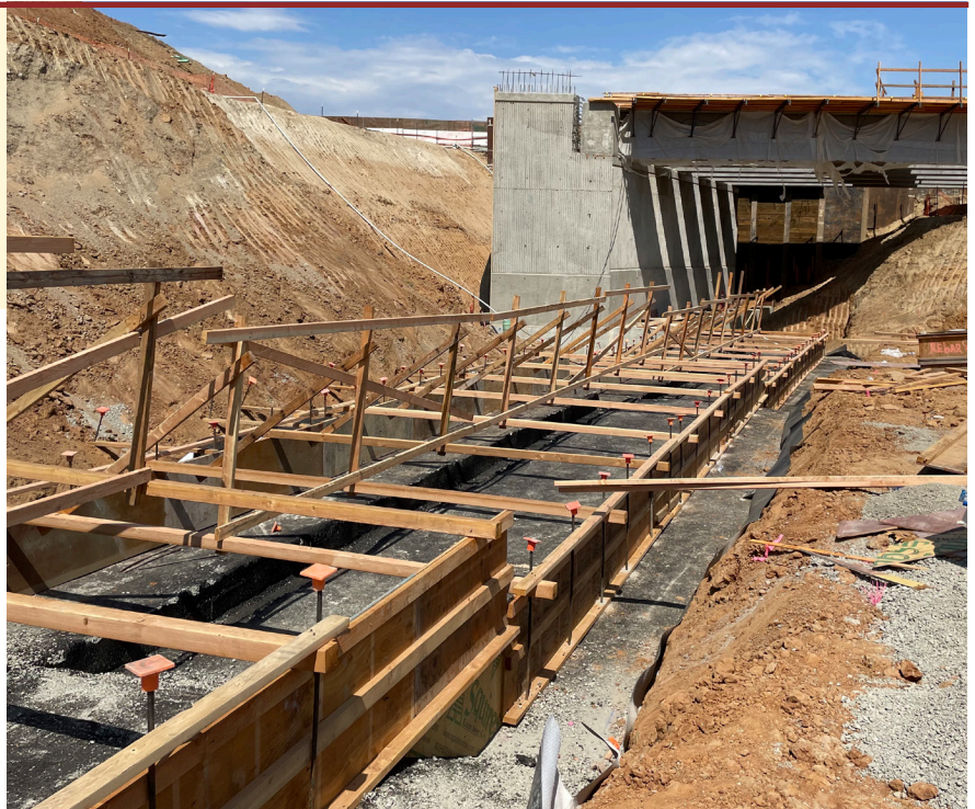
Crews working on the retaining wall support system next to Jurupa Road where it is lowered under the Van Buren Boulevard bridge.
