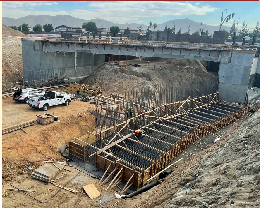
A “behind the k-rail” look at construction on the wall footings where crews will place nearly 500-cubic-yards of concrete early Wednesday morning.
