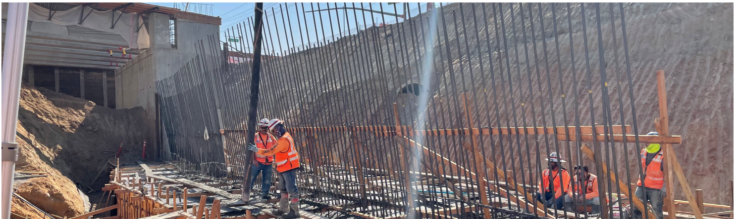
Crews placing concrete for the retaining wall support system where the Jurupa Road west underpass is being constructed.
