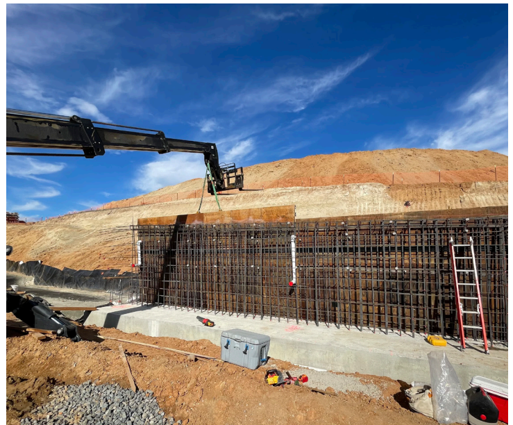
Crews working on the retaining wall support systems for the Jurupa Road underpass.
