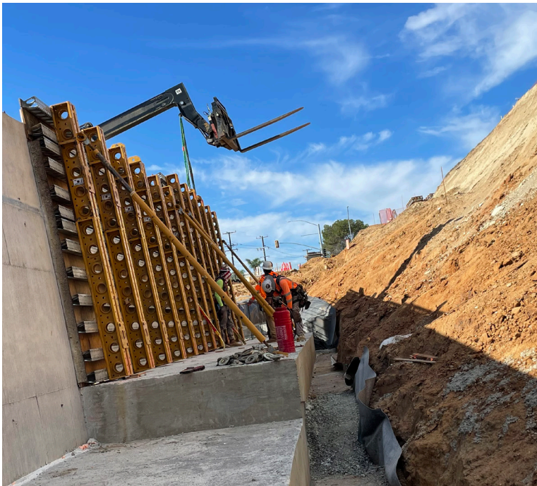
Crews working on the retaining wall support systems for the Jurupa Road underpass.
