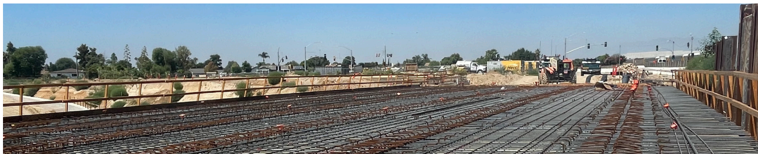
Check out the progress on the Van Buren Blvd. bridge deck.
