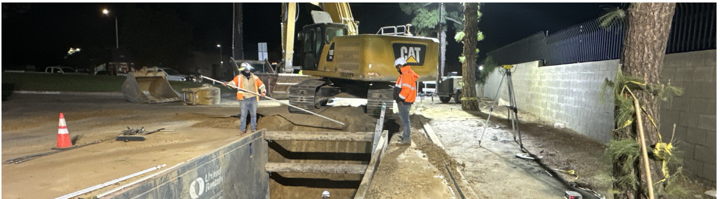
Crews finishing storm drainage installation behind the Stater Bros. last week.
