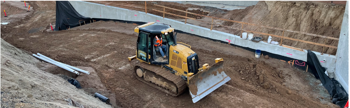
Crews backfilling at the Jurupa Rd. underpass retaining wall system.
