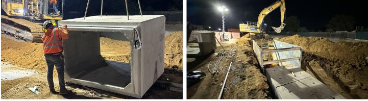
Contractors at work installing the concrete storm drain. They are working in a northwesterly direction to connect the Bly Channel, storm water pump station and the Jurupa undercross systems together to prevent flooding during future storm events.
